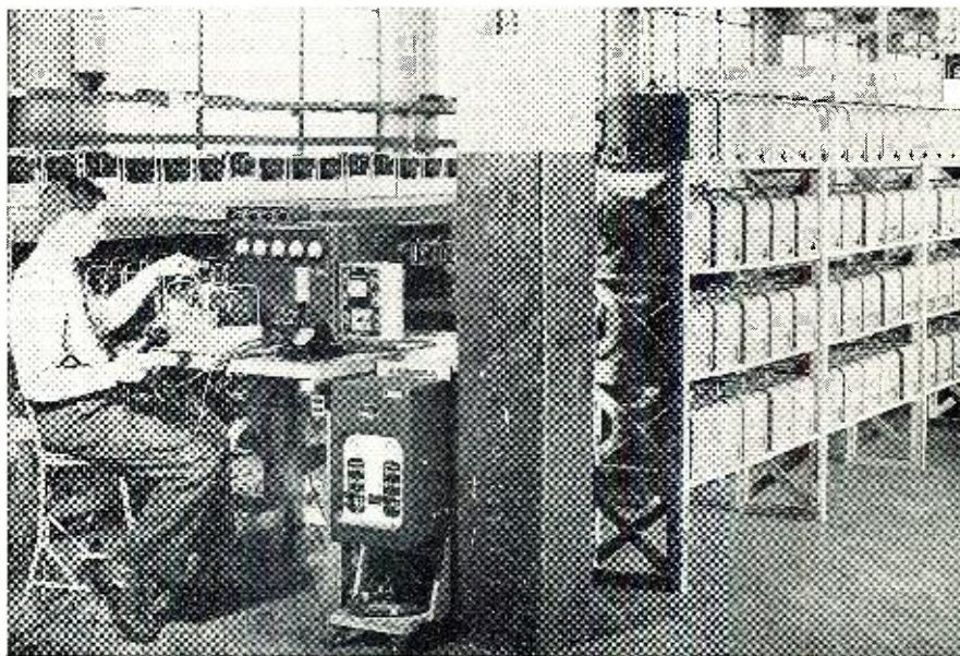
G.E. engineer testing new two-way FM police radio equipment.
